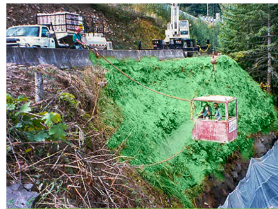
Soil Guard® conforms to the contours of bare soil on contact for immediate erosion control protection. Because it is hydraulically applied, Soil Guard can be used to treat areas that are difficult or impossible to protect with other erosion control systems.
